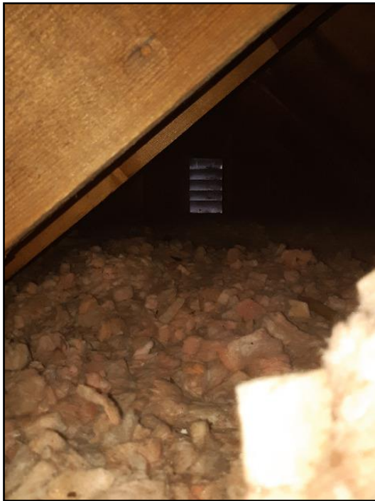
85. Inadequate in knee wall areas
