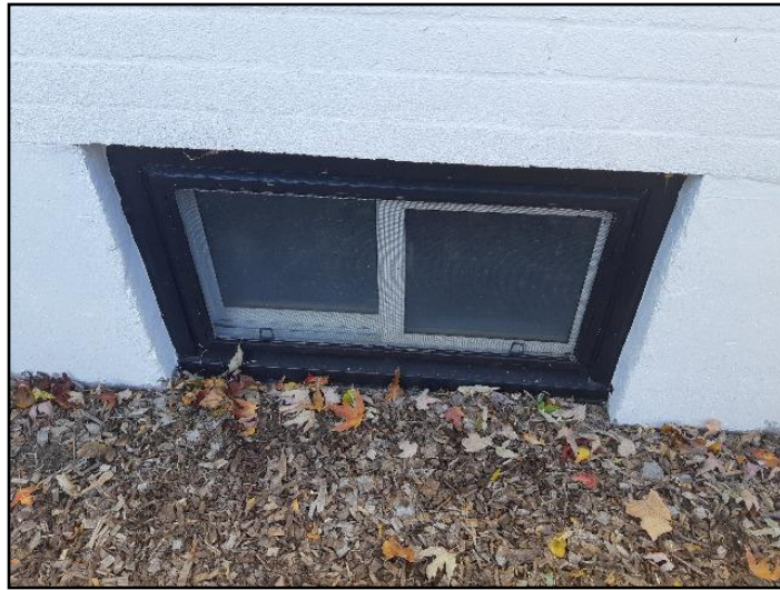
41. Wood/soil contact
